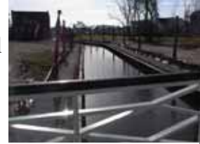
Jefferson Bridge & Towpath # 10
